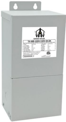
TX-BB-120V-132V-20.8A — NEMA 3R Encapsulated, cETLus Listed
